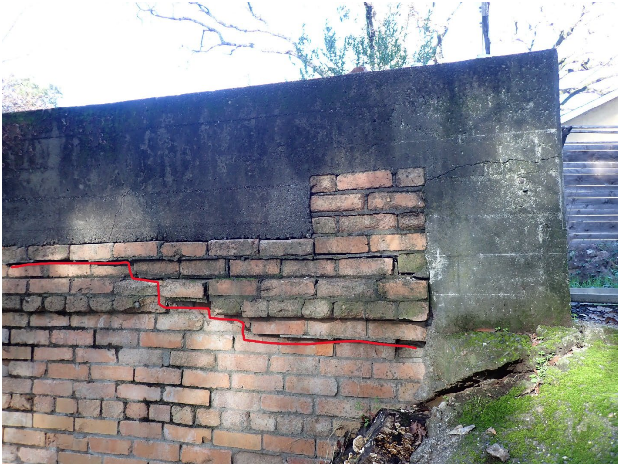
Photo 2 – Headwall damage
