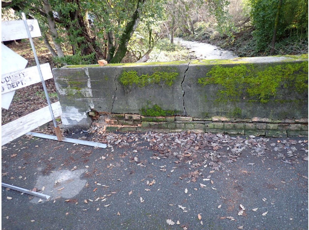
Photo 3 – Rail Damage
